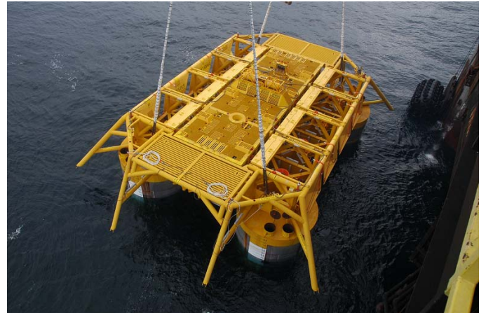
Fig. 8 Installation of Template A
