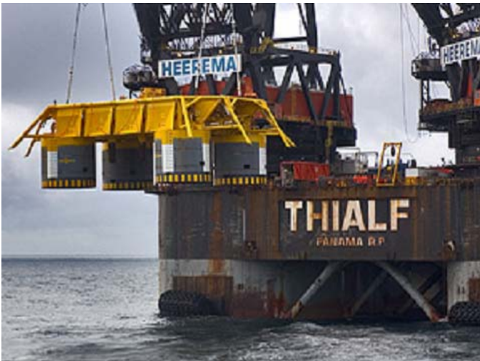
Fig. 7 Installation of template from Thialf
