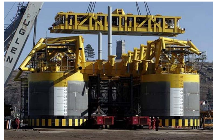
Fig. 5 Lifting of manifold module onto the FBS
