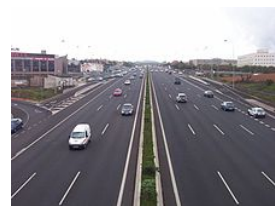
Autopista TF-5 passing by the Guajara Commercial Area and the Central Campus
